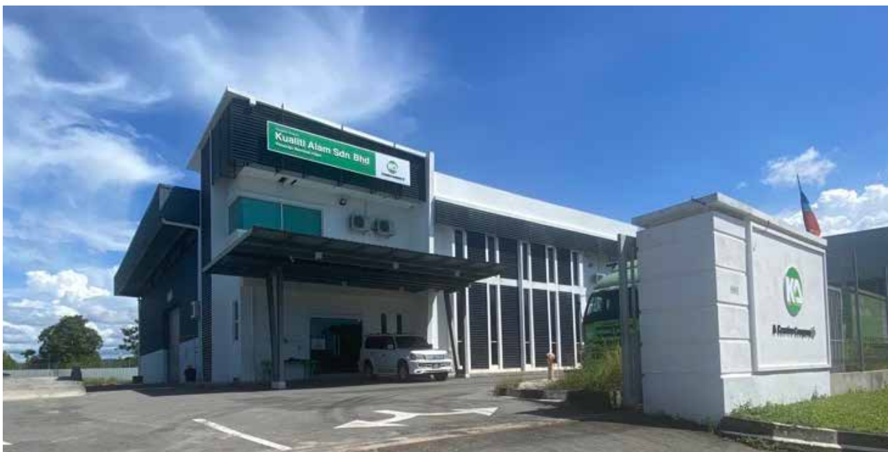
KASB temporary scheduled waste storage facility in Sabah began operations in 2018.
