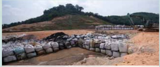
Existing waste used as bund for secured landfill
