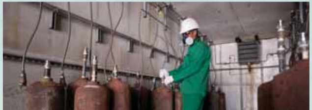
Recovering acetone at the acetylene plant
