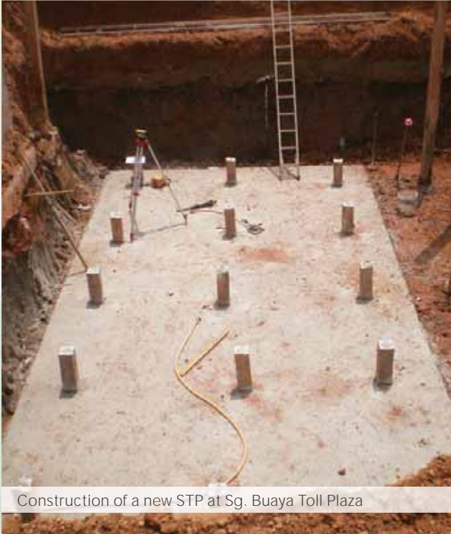
Construction of a pump sump basement slab
