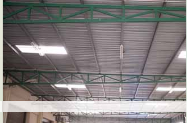
Replacing a normal fluorescent tube with an LED equivalent
