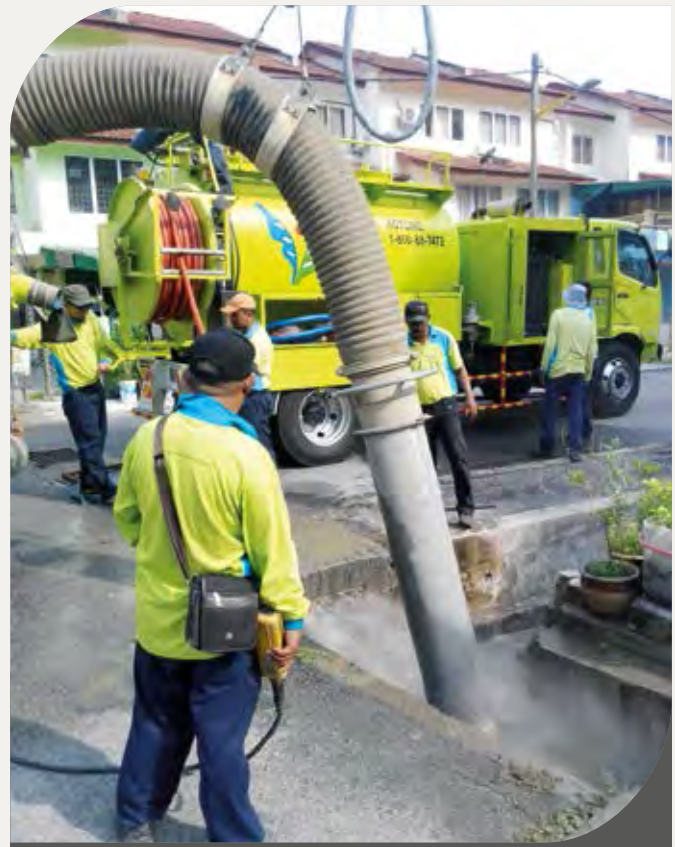
Drain cleansing activities at Pulau Pangkor
